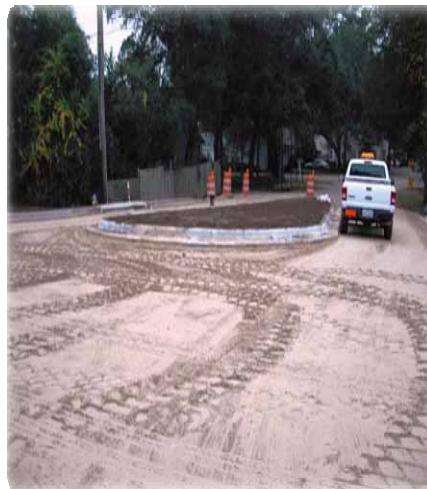
US 90 (Mahan Drive) Buckwood Subdivision Entrance is underway.
