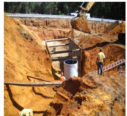
Drainage activities in Segment 1.
