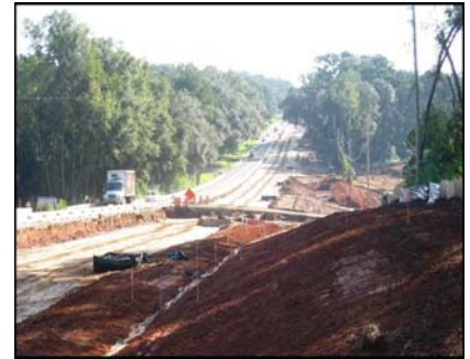
Embankment work on eastbound Mahan Drive just north of Dempsey Mayo.
